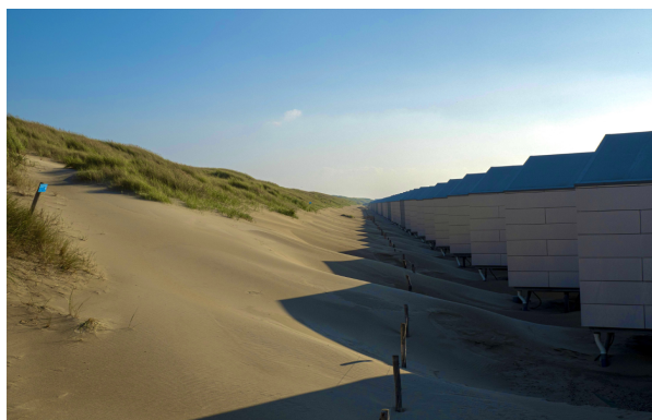
Figure 5.3: A row of closely-spaced vacation houses with deposition regions behind their lee face. The buildings are placed at a close distance to the dunes (photo by Daan Poppema.)
