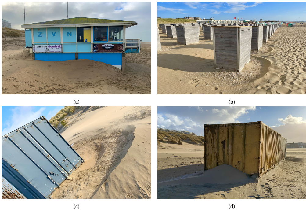
Figure 1.2: Wind-induced morphological patterns around buildings at the beach; a) a restaurant that was buried in sand at Noordwijk beach, the Netherlands, b) a row of small-size beach huts with erosion around at Katwijk beach, the Netherlands, c and d) a container with erosion in front and sand accumulation behind just a few days after it was placed at Noordwijk beach, the Netherlands.
