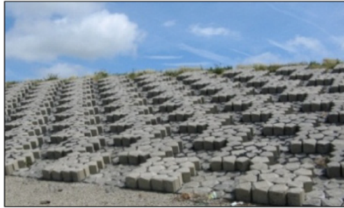
Figure 4.3: Chessboard pattern of Basalton® block revetment (from Capel, 2015).
