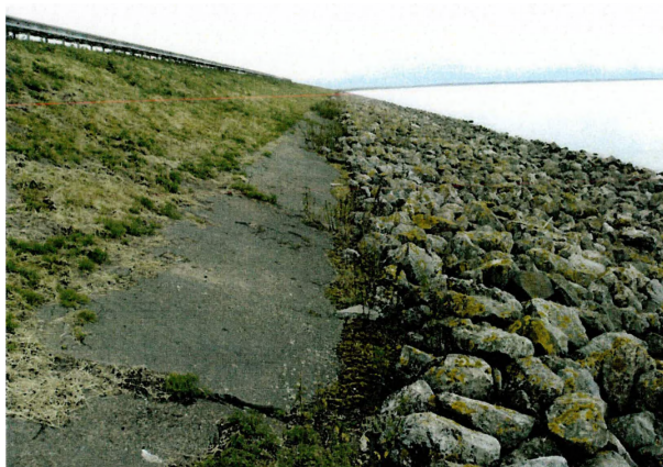
Figure 3.1: Rock armour on the low part of the seaward slope (from Van der Meer, 2004)
