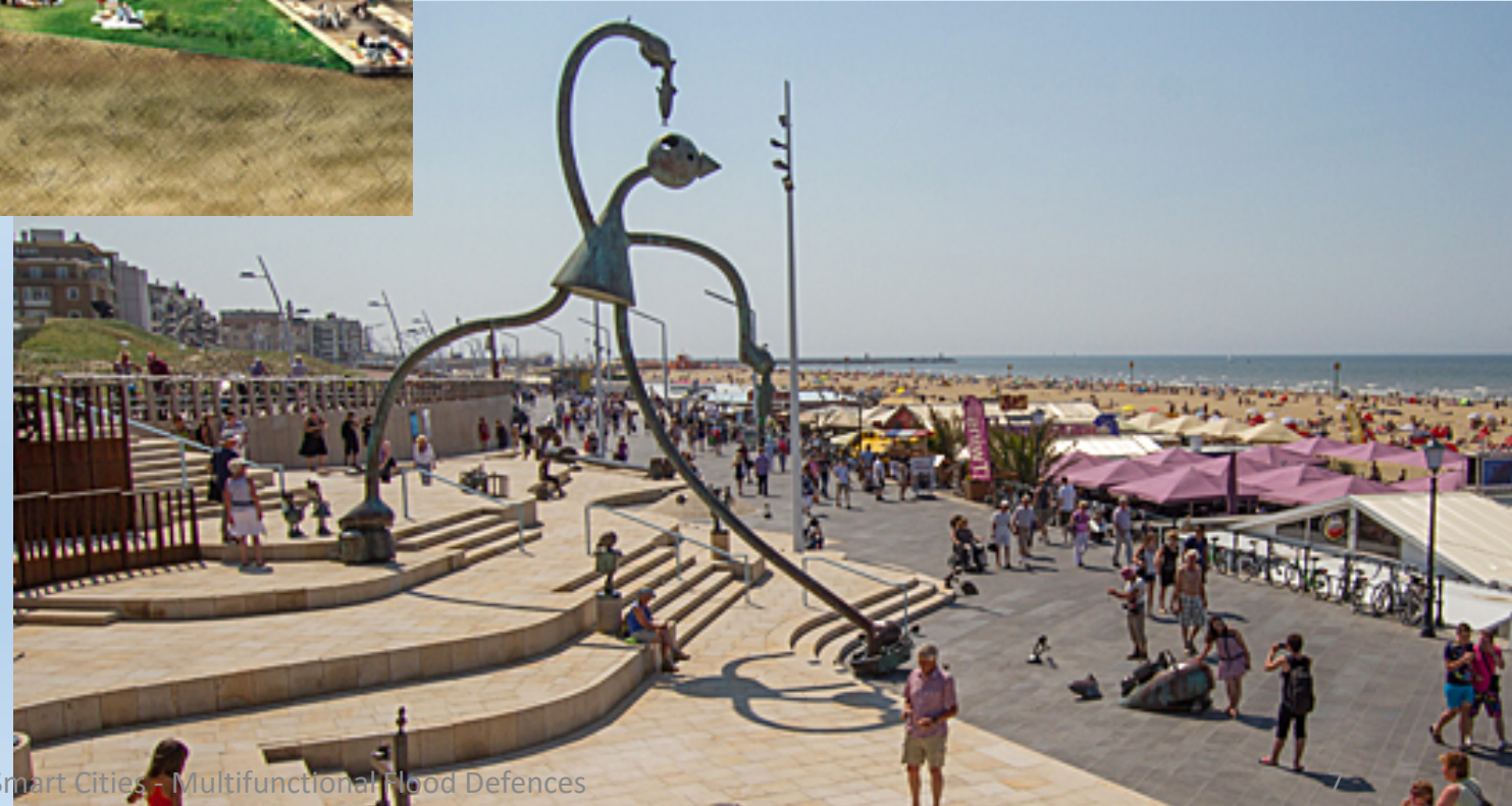
The Hague flood retention wall
