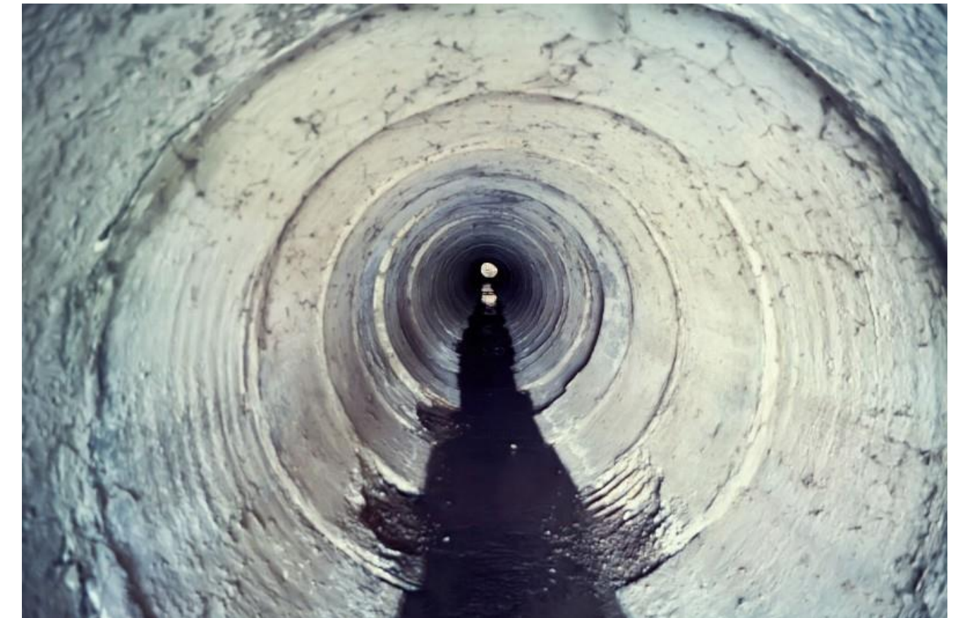
Image retrieved from: https://sunburstev.com/drain-line-camera-inspection-cctv-technology/
