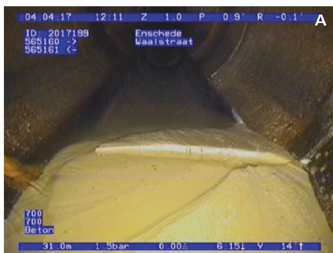
Figure 3. a) CCTV image acquired by the Municipality of Enschede, it can be clearly seen infiltration of sediment from the road into the sewer pipe. b) Optical image acquired with optical game camera Moultrie m-series showing the test site in Waalstraat. Notice the deformation on the road (red circle) caused by infiltration of sediment into the sewer pipe. c) Thermal infrared image acquired on February 15 2020 at 16:15 hours.
