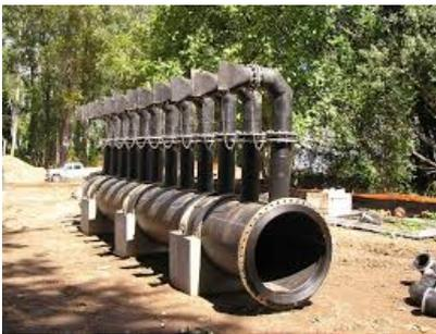
Figure 3.6: Example of a diffuser outfall pipe (Doneker, 2014)
