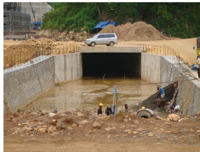
Figure 3.7: Example of surface port outfall system (PembangkitListrik, 2015)
