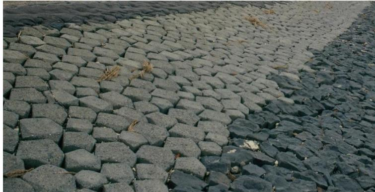
Appendix figure 3 Placed blocks (basalton) bed protection (Rijkswaterstaat, 2015)
