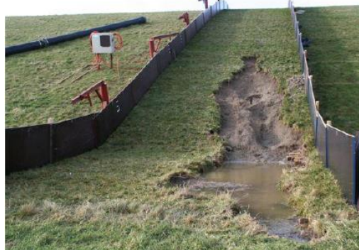
Figure 1: Example of grass cover erosion at the landward toe after a test with the wave overtopping simulator (Van der Meer, 2014)
