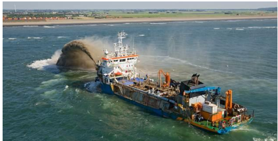
Figure 1: Application of shoreface nourishment near Callantsoog (Rijkswaterstaat, 2017)
