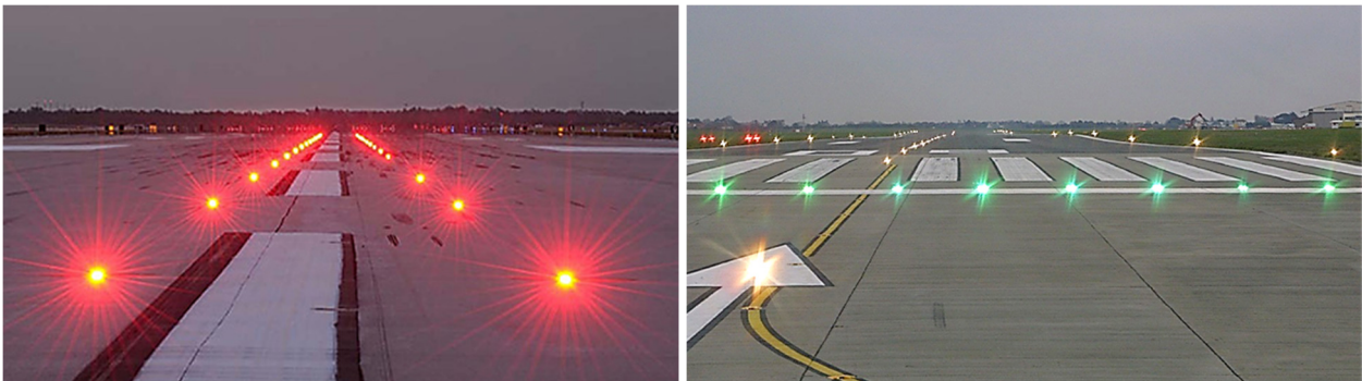
Figure 2-3: Take-off Hold Lights (left) and Runway Threshold Lights with an aligned taxiway (right)
