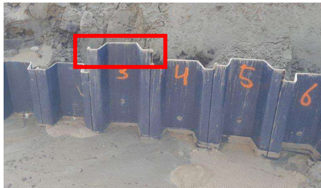
Figure 21. Incorrectly installed sheet pile at project Wolferen Sprok (red box: sheet pile not at required depth).
