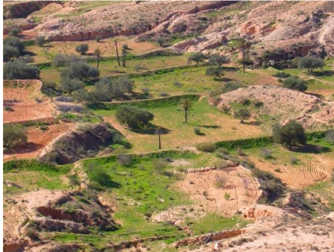
Figure 52 - Example of small dams on a slope
