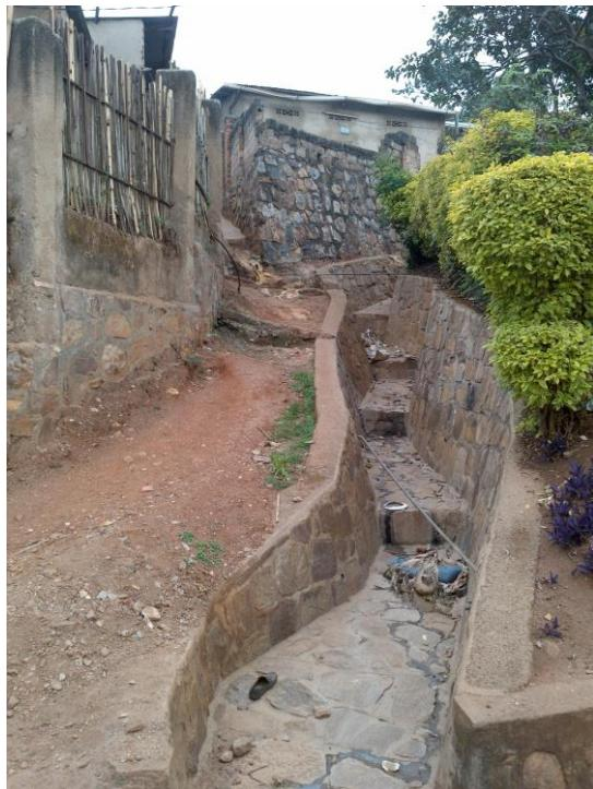
*Figure I- 1 – stepped drain in Mpazi*
