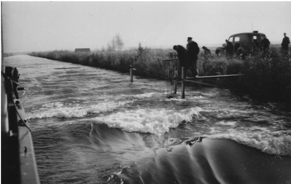
Figure 2.1: Measurements of squat being done for Schijf (1949).
