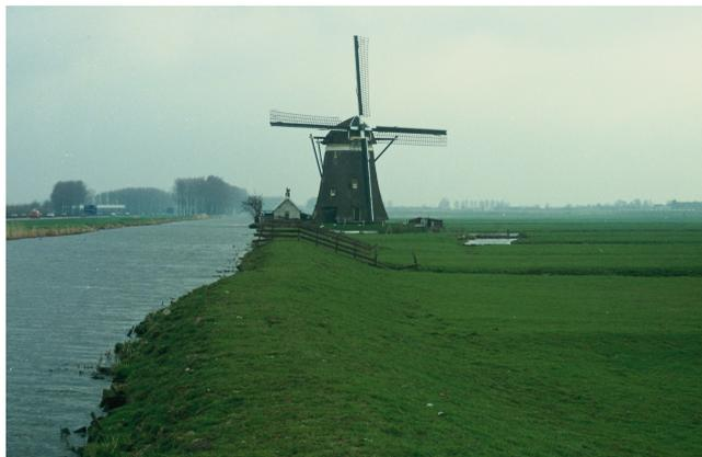
Figure 1.1: A canal dike example for which ship waves can be normative for overtopping.
