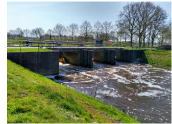
Figure 1: Weir in the Dinkel River. Note the natural flow seeding (foam) due to the interaction between the water and weir.
