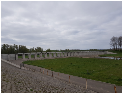
(a) Pannerden, located in the floodplain of the Pannerdensch Kanaal just downstream of the Pannerdensche Kop bifurcation. The picture shows the structure with nearly all beams removed. Photo: Matthijs Gensen
