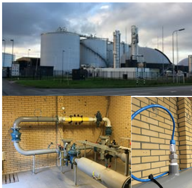
Figure 4: Sugar biogas plant in Groningen, and gas sensor installed in Gas Distribution Station.
