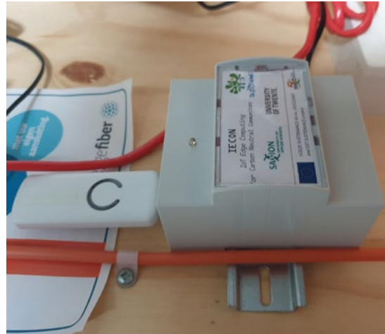
Fig. 1 IECON system installed at Vriendenerf
