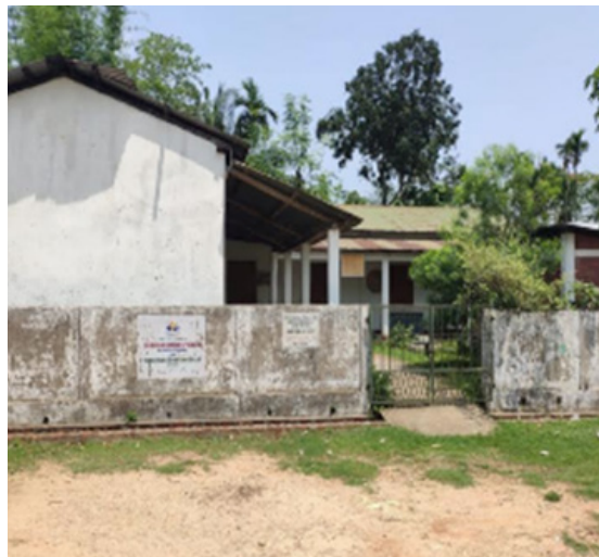
Case 2: BORAKHAI VILLAGE, which aims at delivering smart clusters based on local energy systems powered by renewables
