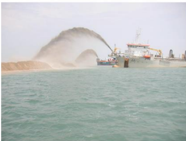
Figure 6.9 Bund construction using rainbowing.
