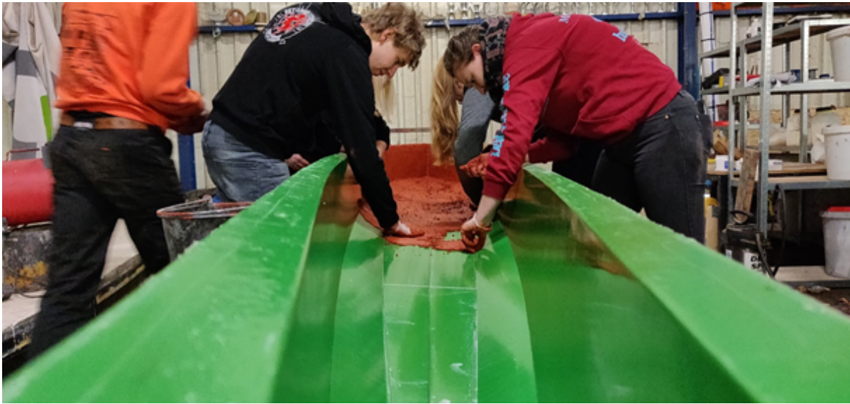
Figure 4: Applying the first layer of concrete to the mould.
