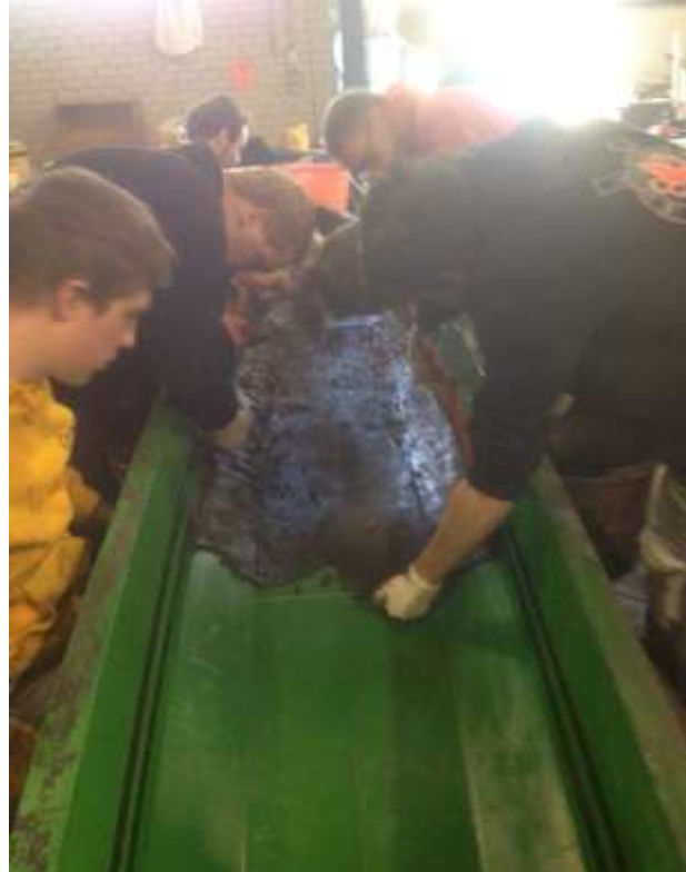
Figure 19: applying the concrete to the canoe
