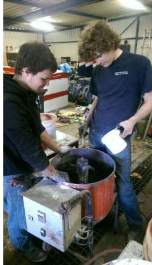
Figure 15: Brewing the concrete at the construction site
