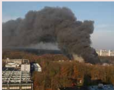
THE FIRE IN THE TW/RC BUILDING 2002
