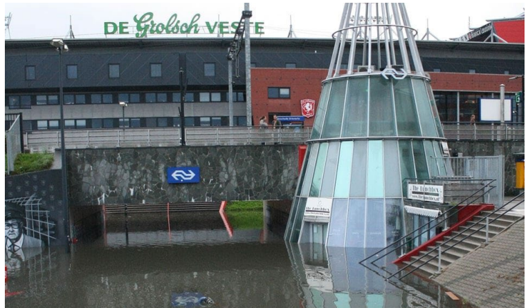
Figure 1: Underpass Enschede Kennispark flooded.
