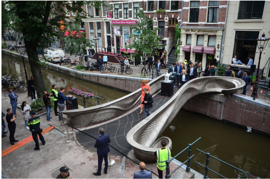
MX3D Bridge Amsterdam
