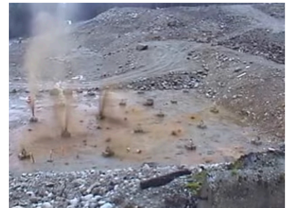
Fig 1: (Top) schematic of the explosive compaction, courtesy of Menard ; (Bottom) soil spreading and water rise after blast explosions.
