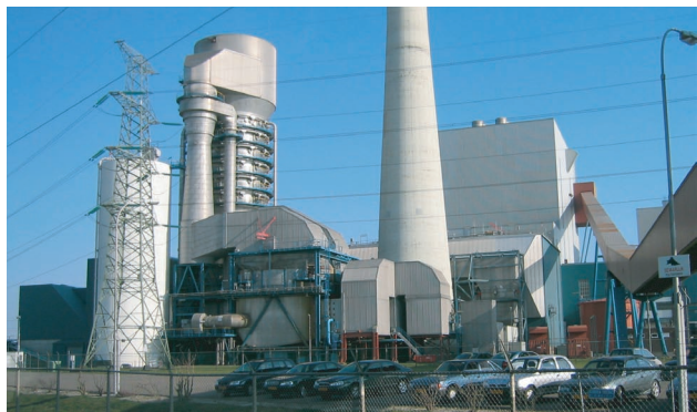
Figure 4: Coal fired power plant (Borssele, The Netherlands).
