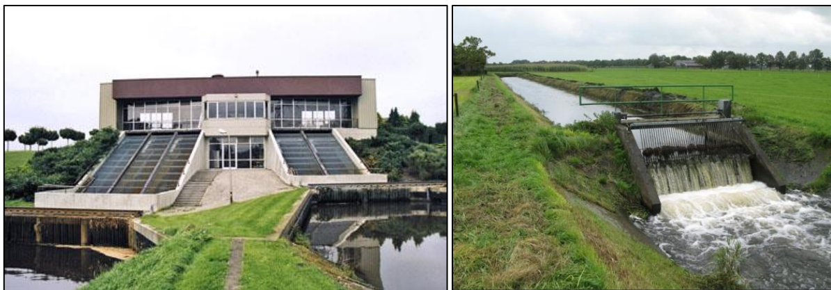
Figure 4-1 Pumping station 'Nieuw Lutterzijl' (left) and an example of a weir (right)
