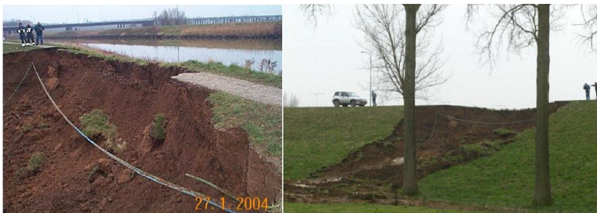
Figure 3; Dike failure at Stein (van Vollenhoven et al., 2005)
