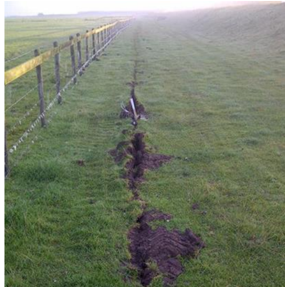
Figure 68; Pipe/cable located next to dike (Hoogheemraadschap De Stichtse Rijnlanden, 2010)
