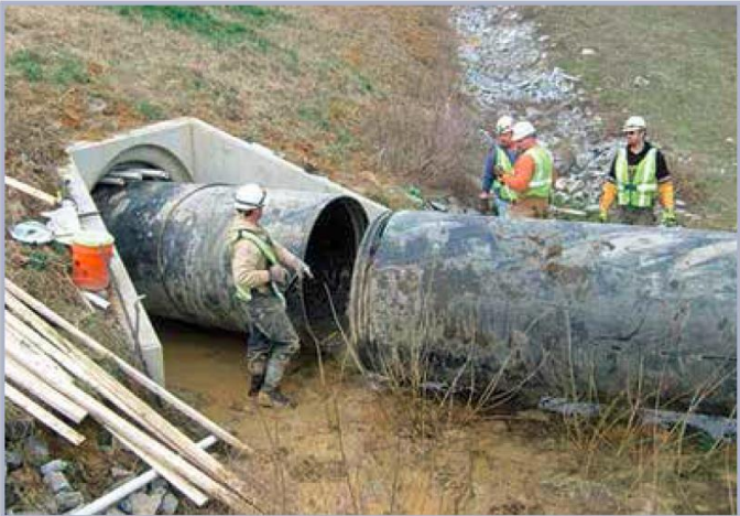
Figure 6; Installation of buried pipe in embankment (David Pezza & Hal Van Aller, 2005)
