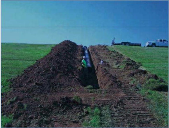
Figure 5; Pipeline on top of dike (Finsbury et al., 2013)
