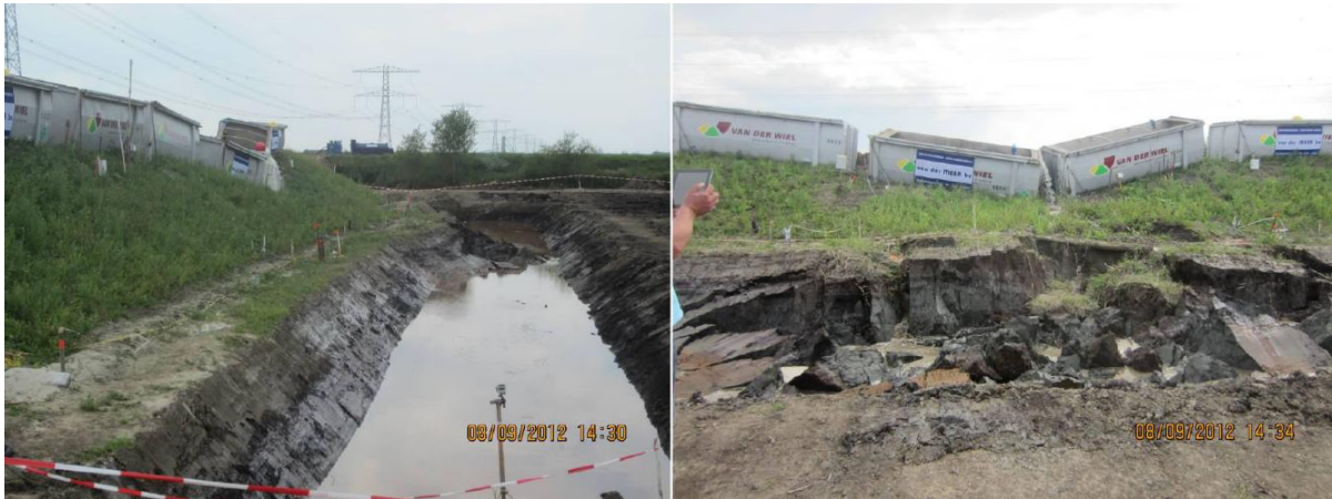
Figure 16 Failure of South dike (Vries et al., 2012)
