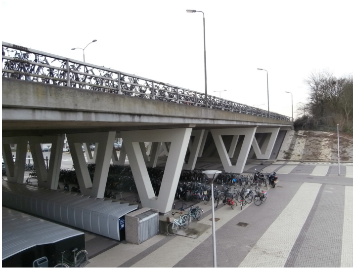
Figure 7.15: Delft South bicycle parking facilities (University of Twente - LUTI students field work, 2013)
