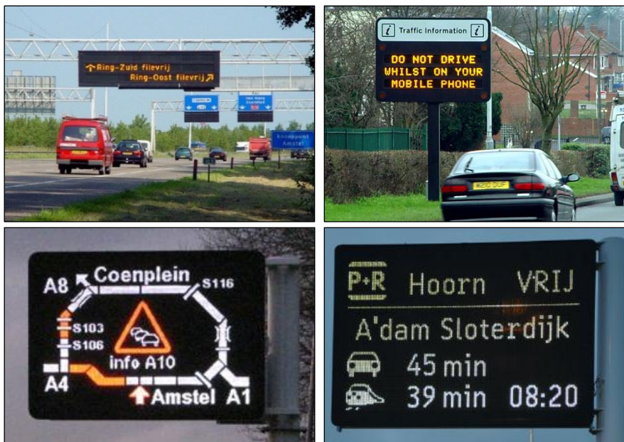
Figure 3 Mono-coloured VMS with text: congestion information (top left) and campaign information (top right). Duo-coloured VMS with text and graphics: congestion information (bottom left) and travel times of public transport and car (bottom right)
