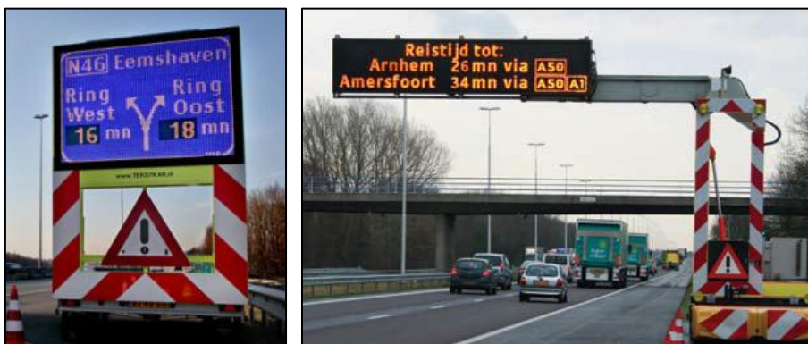
Figure 92 Travel time information on VMS on rural road (left) and freeway (right) operated by VID (VID, n.d. d)
